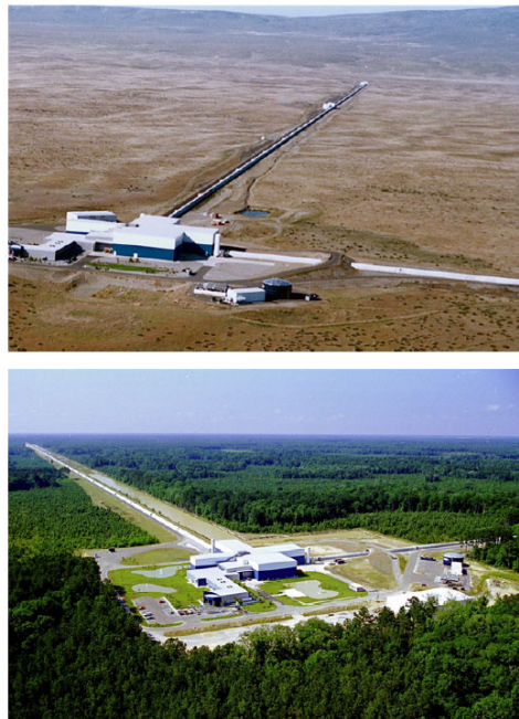
Figure 2. Aerial photograph of the LIGO observatories at Hanford, Washington (top) and Livingston, Louisiana (bottom). The lasers and optics are contained in the large corner buildings. From each corner building, evacuated beam tubes extend at right angles for 4 km in each direction (the full length of only one of the arms is seen in each photo); the tubes are covered by the arched, concrete enclosures seen here.
